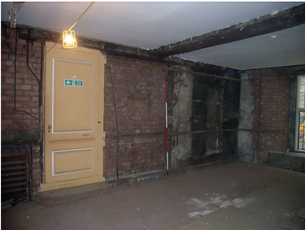
Fig. 2. The east wall of the Eckersley Room after removal of twentieth-century panelling, showing the painted panel in situ.
